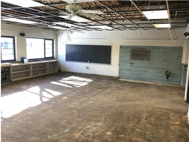
MacGowan Elementary School - Classroom Demo
